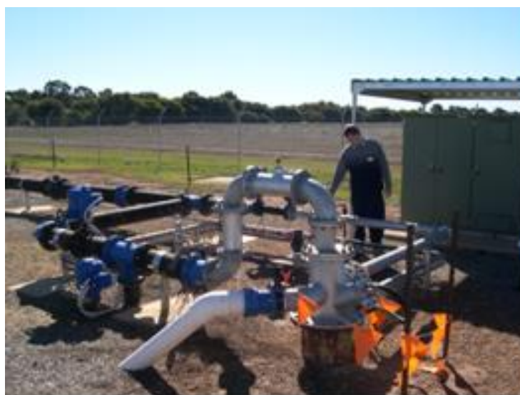
Figure 6. An aquifer storage and recovery well to inject wetland-treated stormwater into a brackish limestone aquifer for recovery in summer for irrigation around the city of Salisbury, South Australia (photo: P. Dillon).
