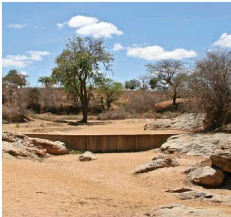
Figure 3. Sand storage dam in good condition (photo: Acacia Water).
