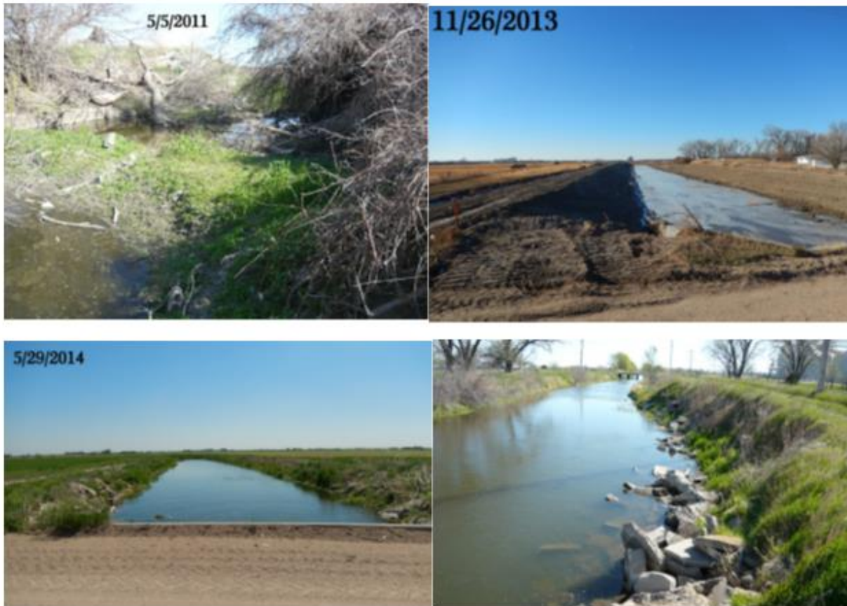
Figure 2. Overgrown canal in disrepair (upper left), canal after grading and clearing (upper right), canal section after project completion (lower left) and headworks of the canal after project completion (photos: CPNRD [6] ).
