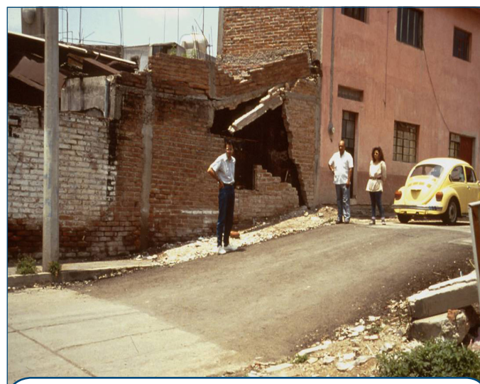
MAJOR LAND SUBSIDENCE IN RURAL MEXICAN TOWN RESULTING FROM EXCESSIVE WATERWELL ABSTRACTION
