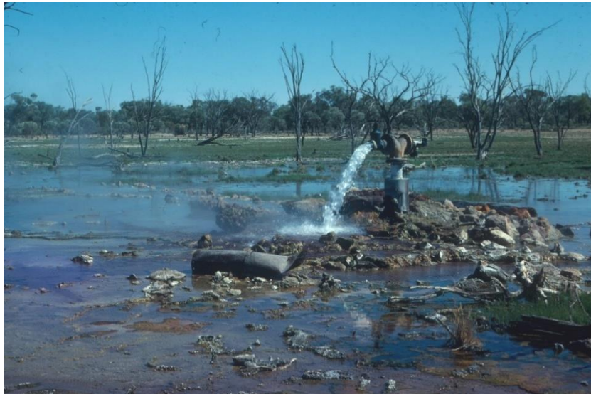
Figure 2. The Great Artesian Basin, Australia – Uncontrolled flowing artesian water bore (photo: M. A. Habermehl).
