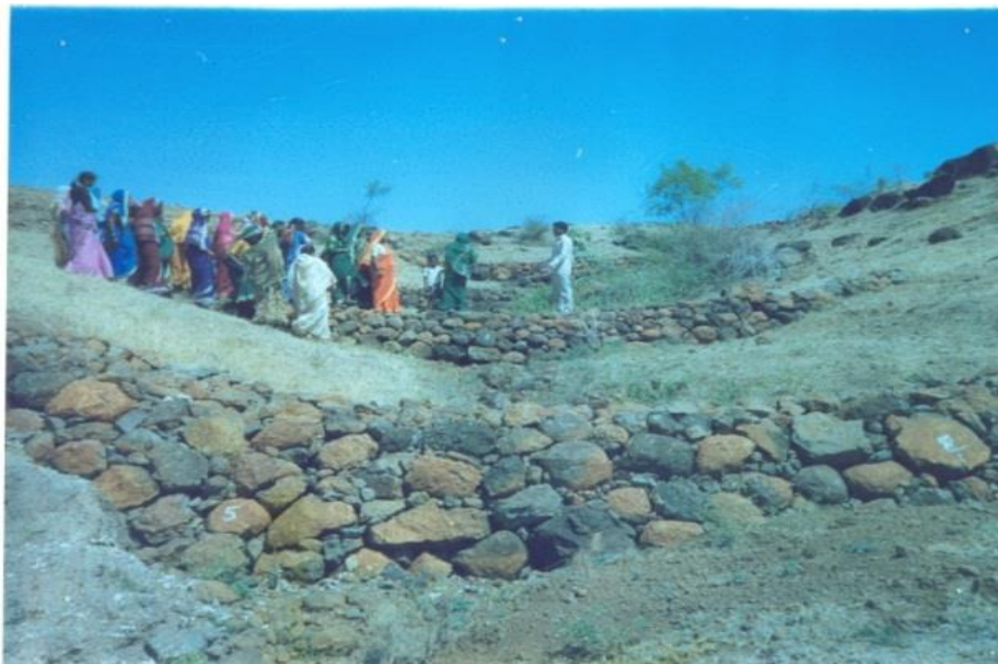
Figure 2. Lose boulder check dam (photo: Kadwanchi project implementers).
