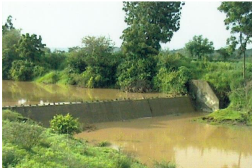
Figure 3. Water harvesting check dam (photo: A. Sikka).
