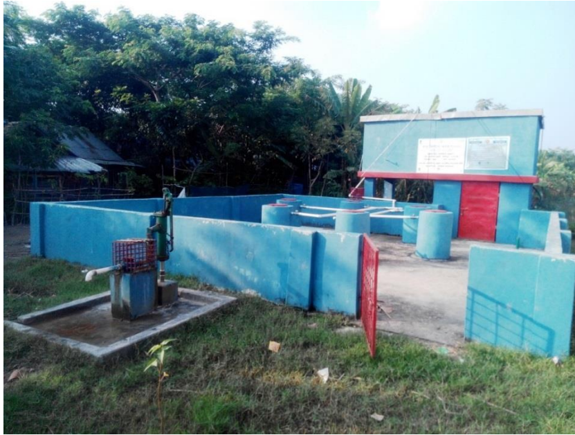
Figure 2. A typical MAR system showing various components (photo: Riyadul Islam).
