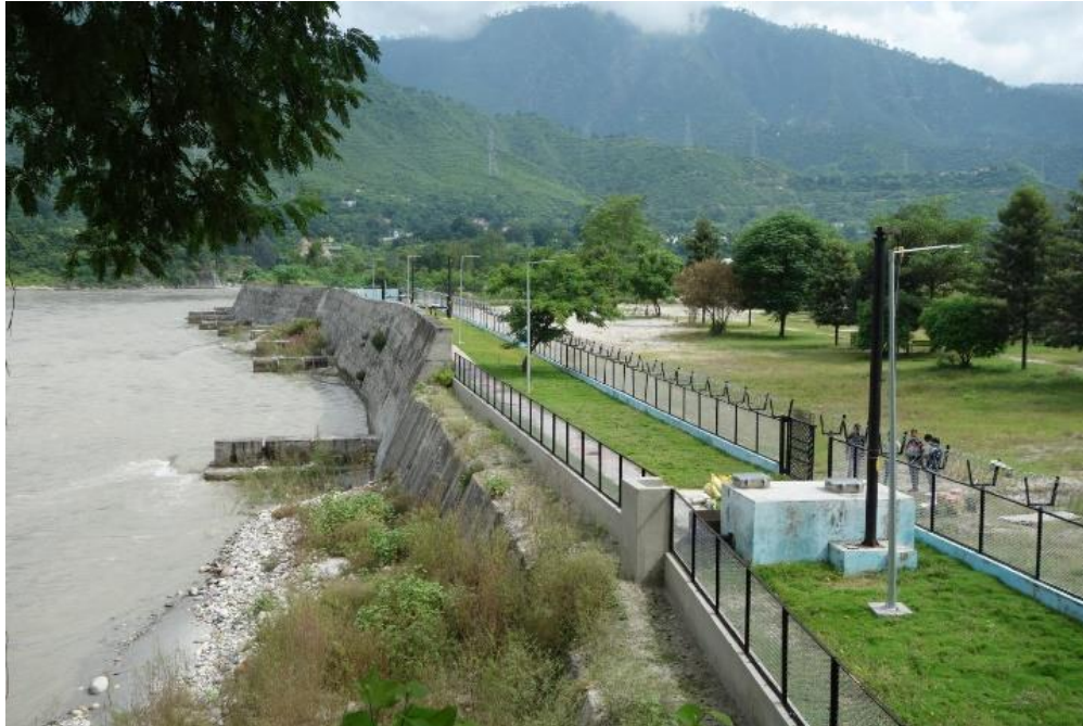
Figure 4. RBF well equipped with a flood-proof well chamber and a watertight wellhead (photo: HTWD).
