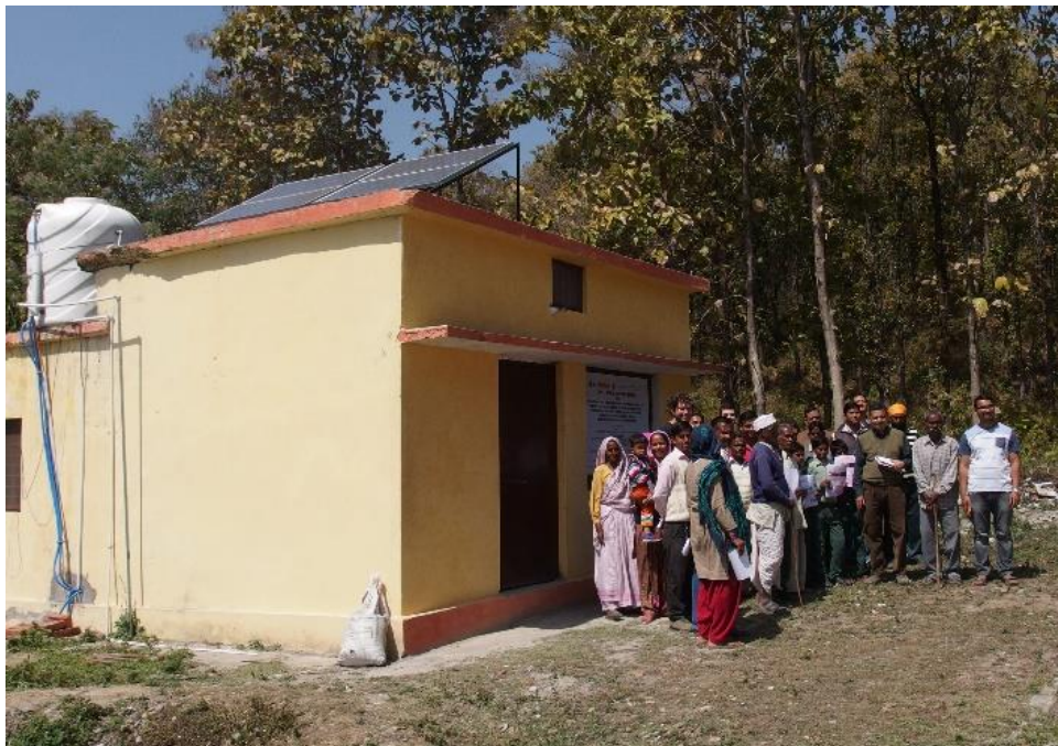
Figure 2. Workshop to create awareness of disinfection by photovoltaic (solar) powered small-capacity inline-electrolysis disinfection systems at an RBF site in Julo village, Uttarakhand (photo: P. Otter/AUTARCON).
