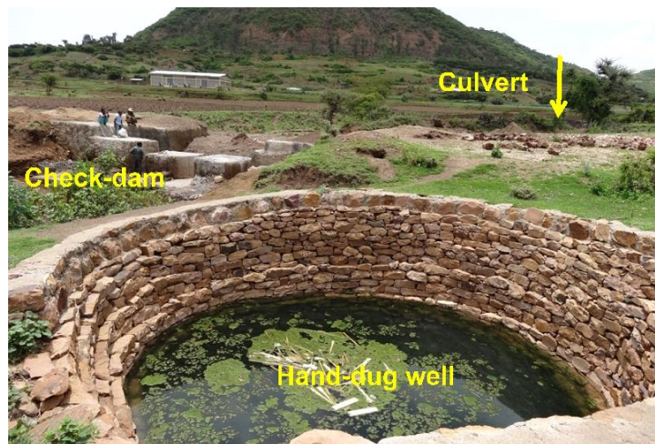
Figure 3. Check dam downstream of culvert retaining water and recharging hand-dug well (photo: K. Woldearegay).
