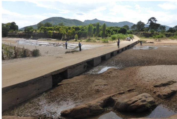
Figure 4. Road crossing acting as a sand dam retaining water upstream in Kenya (photo: MetaMeta).
