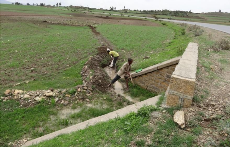
Figure 1. Water diverted from culvert to percolation pond for groundwater recharge (photo: K. Woldearegay).
