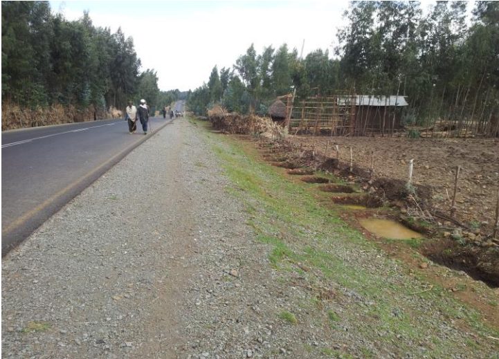
Figure 2. Roadside trenches in Ethiopia (photo: MetaMeta).
